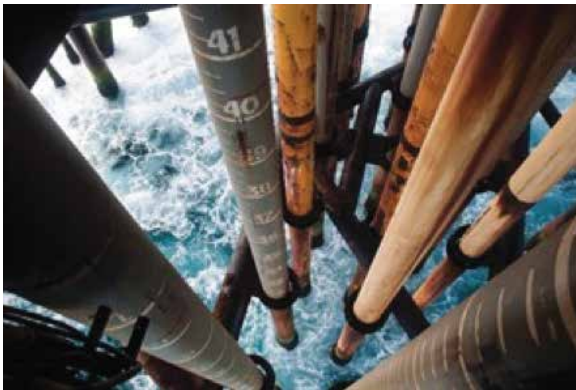
Figure 1: Corrosion monitored on conductors of well head towers (left), illustration of risk based remaining life (right)
